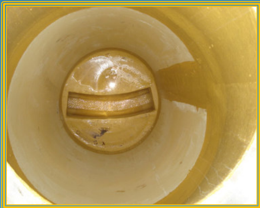
Rehabilitation with GRP base-liner + GRP shaft lining 3 mm
