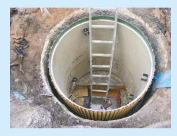
The cover-slab (or cone) is also lined with PP in order to assure a continious and durable air tightness to the rehabilitated manhole which will have a live time equal to a newly built manhole.
