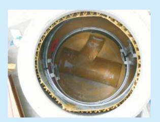
A particular advantage of this system is the flexibility of the polypropylene liner which allows the rehabilitation work even when the cover slab or cone can not be removed.
