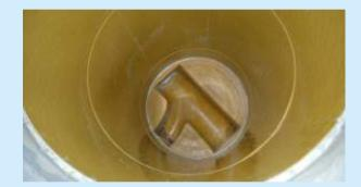
Parallel to this system, the classical PREDL® manhole lining is still available for the manhole rehabilitation. Instead of the PP liner, a GFRP in-liner is used and fitted on a manhole base-liner. The existing manhole structure is also lined to the desired height and the joints are laminated in order to assure a complete water and air tightness. The gap between the manhole ring and the GFRP is also filled with liquid mortar.
