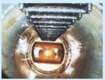
Conclusion: Both rehabilitation solutions can be performed in a relative short time. Using PREDL® PP liners for the manhole ring allows the rehabilitation of open manholes as well as the rehabilitation of manholes "trough the cover-slab or cone". The sewer can be put back in use shortly after finishing the rehabilitation work. The old manhole wall is durably protected against the sewage with the joint free PP/GFRP liner.
