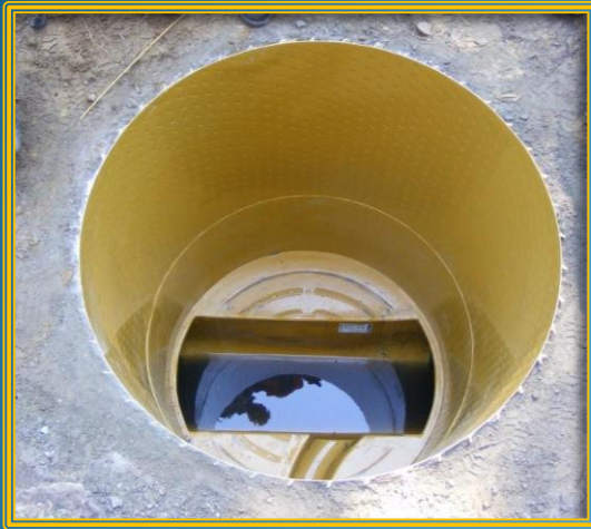
Rehabilitation with CORPROTECT PP lining (coverslab off or through entry hole)
