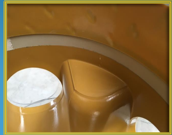
Rehabilitation with GRP base-liner + CORPROTECT liner
