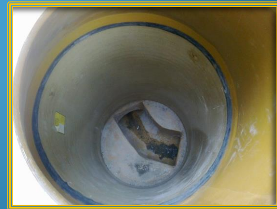
Manhole in manhole solution with GRP manhole base + GRP pipe
