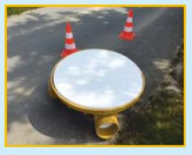
The Styrofoam model is being used as a strengthening for the FLEXLINER when pouring the grout in the manhole base. The Styrofoam strengthening can be delivered in 2 pieces in order to pass through the manhole access hole.
