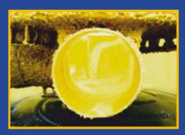
Several solutions are available for connecting sewer pipes or rehabilitation pipe lining: short GRP pipe sockets for GRP pipe liner (wall thickness requested in order to avoid any step in the socket) to be laminated together in the transition area or to be welded to the transition strip with thermoplastic sewer pipes.
