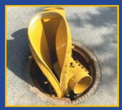
PREDL-FLEXLINERS are made out of chemical resistant Polyruea and can be installed in the manhole in one piece, without having to be cut up.
